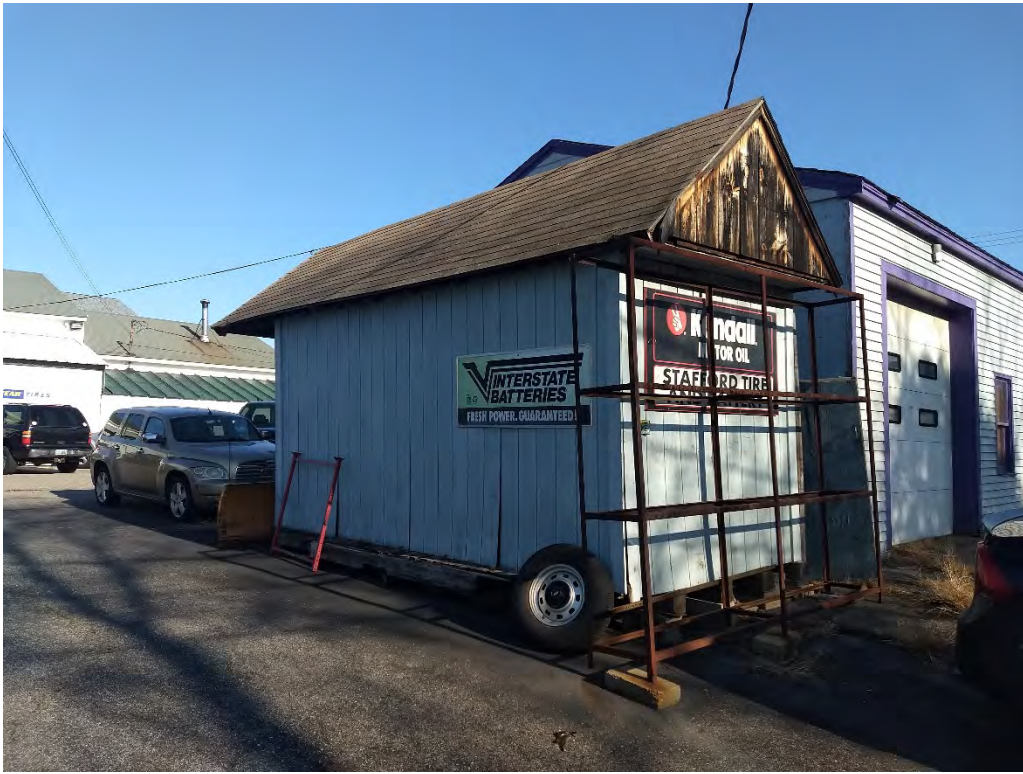
Storage shed on north side of #116 Broadway.
