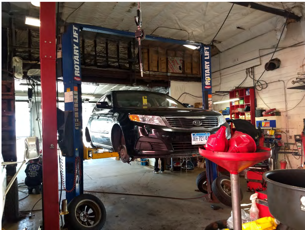
Aboveground floor lift with waste oil collection device.
