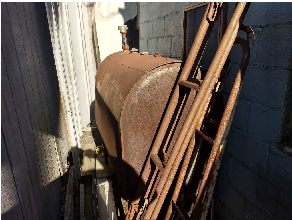
Empty 275-gallon aboveground storage tank on north side of #116 Broadway.
