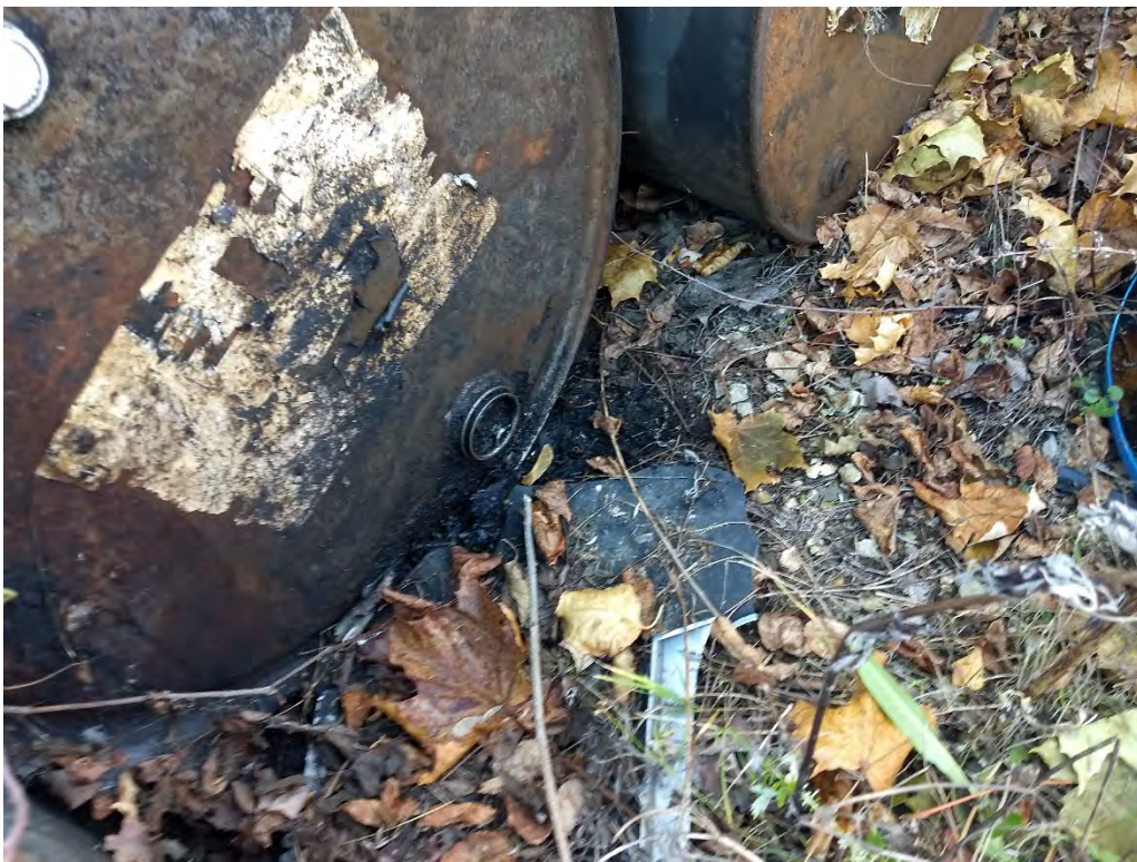
Minor staining adjacent to 55-gallon drum on north side of 118 Broadway building.
