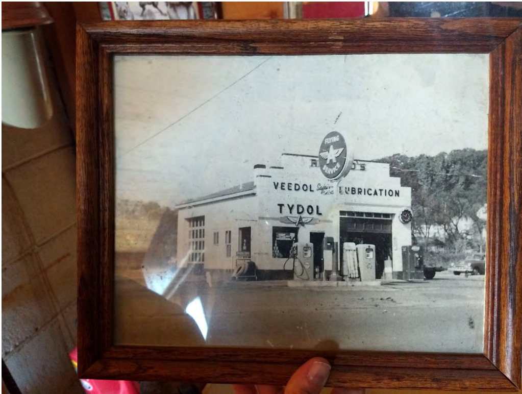
Photograph of old gas station at Site.
