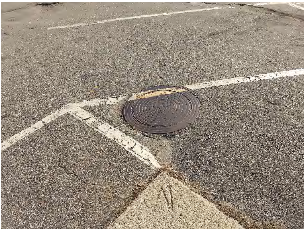
Manhole cover on south side of 118 Broadway building.
